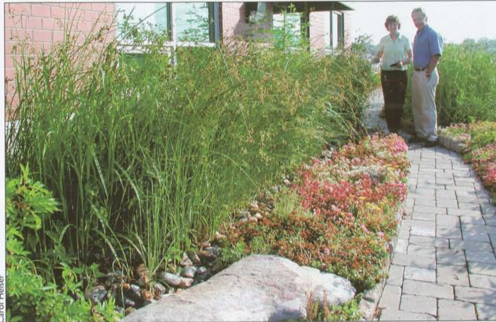
Wetland Studies and Solutions, Inc. in Gainesville is an exemplary model of corporate habitat success. The green roof seen here captures and treats rainwater, which significantly reduces the amount of runoff entering nearby creeks. The site also boasts a bioretention swale and permeable paving, all designed to get water back into the ground.
