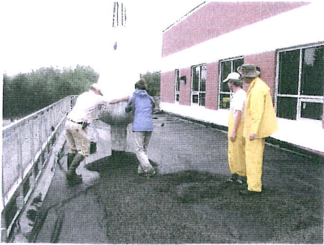
A growing medium was lifted to the green roof by crane.
