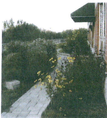
Office building with green roof
