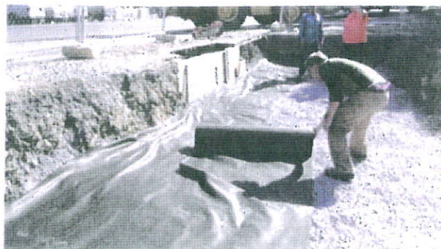
Applying geotextile fabric to floor of rain garden
