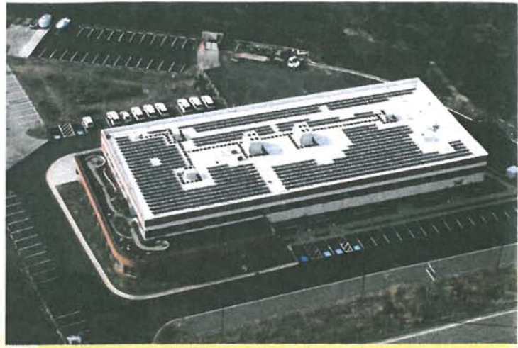
Solar panels nearly fill the roof of the WSSI office building on Wellington Branch Drive in Gainesville. Also note the green roof space on the left side of the building.
