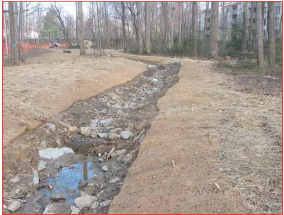
Snakedon Branch post construction: channel is raised to provide floodplain access.
