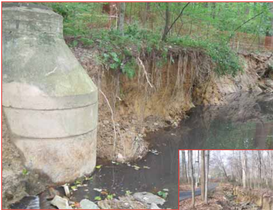
Exposed sanitary manhole within the project area. Inset: Snakedon Branch before: channel is incised and disconnected floodplain.
