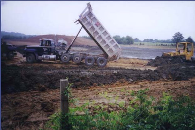
Delivering the Clay Liner Material
