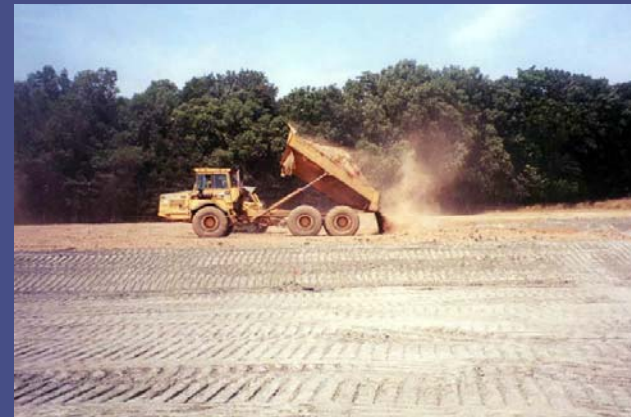
Spreading Topsoil on Clay Liner
