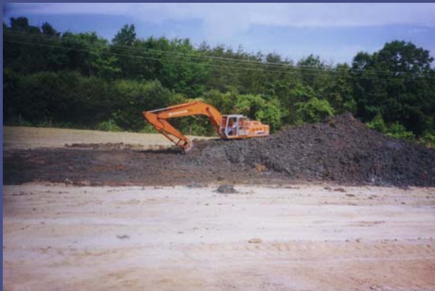
Stockpiling Clay Liner Material
