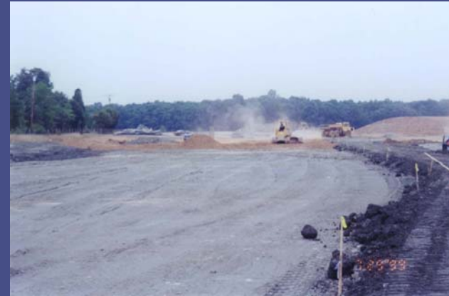
Construction of the Clay Liner
