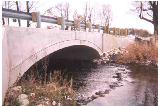
MINOR– Con/Span causing only temporary impacts to Waters of the U.S.
