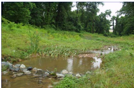
RF = 8.50: Northern Virginia, Urban/suburban stream restored utilizing Natural Channel Design techniques, bed reinforcement, and grade control structures.
