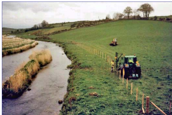
RF=0.25: Livestock exclusion fence placed along the stream to protect the streambanks and riparian vegetation.
