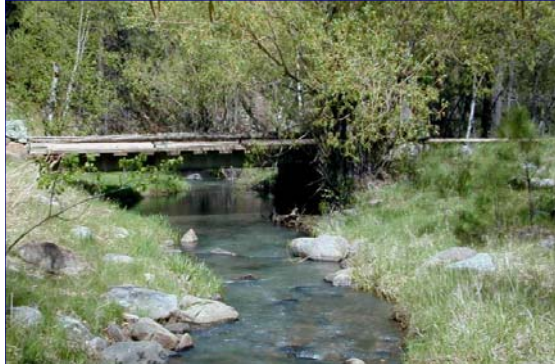
Amenities: Pedestrian bridge placed across a rural stream.
