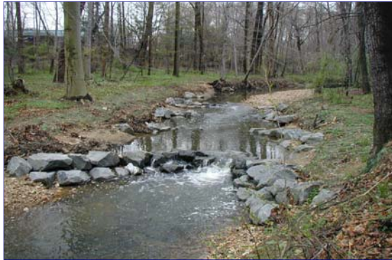
RF = 7.00: Northern Virginia, Urban/suburban stream restored utilizing Natural Channel Design techniques and grade control structures.
