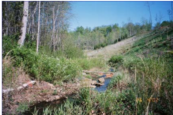
RF = 4.50: Central Virginia, Urban/suburban stream relocated and restored utilizing bioengineering techniques.
