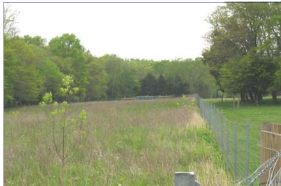
RF = 1.25: Northern Virginia, Installation of livestock fencing and removal of non-native species, deep-disked, seeded and planted native trees and shrubs.
