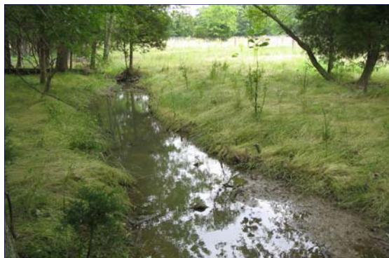
RF = 2.00: Northern Virginia, Rural stream with both banks stabilized utilizing bioengineering techniques. Coir logs are present along the toe of both banks.
