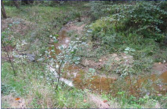
RF = 2.25: Northern Virginia, Urban/suburban stream utilizing bio-engineering techniques on one bank. The left bank was regraded with biologs placed at the toe of the slope and the bank was replanted with native vegetation.
