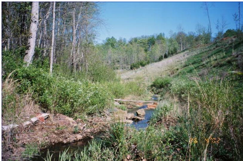
RESTORATION 2 - Bioengineering and relocation of an Urban/suburban stream.
