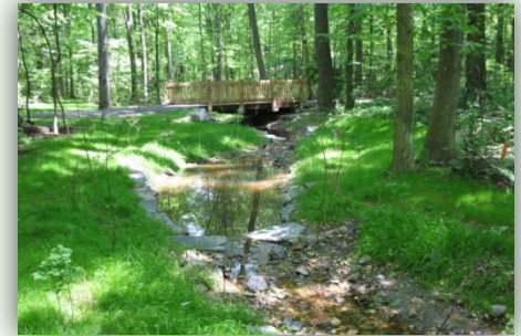
Restored conveyance system
