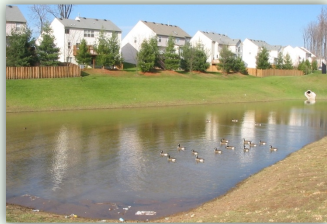
Extended detention pond
