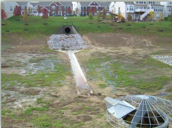
Extended detention pond
