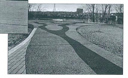
What is Pervious Concrete? In simplest terms, Pervious Concrete is a mix of coarse aggregate, cement, water, and little to no sand. The addition of certain chemical admixtures can enhance the properties of the Pervious Concrete mix and assist in placement. Also known as "no-fines" concrete, this mixture creates an open-cell structure allowing water to filter through to the underlying soil.
