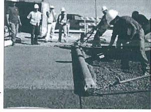
instructs contractors on the properties of pervious concrete and the proper installation techniques. Many of the specifications being written currently require NRMCA Pervious Concrete Contractor Certification as a prerequisite.
