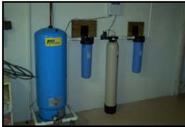
Fig. 15: Residential UV light potable water treatment Photo courtesy of Rainwater Management Solutions
