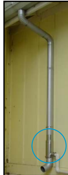
Fig. 9: Downspout filter
