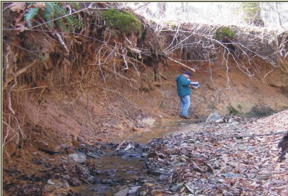
Eroding meander bed adjacent to a roadway
