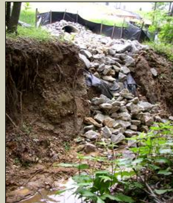
Newly installed outfall into a recently incised channel
