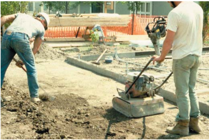
Fig. 1.15 Typical construction environment where compaction and construction activities create difficult conditions for post construction landscapes.
