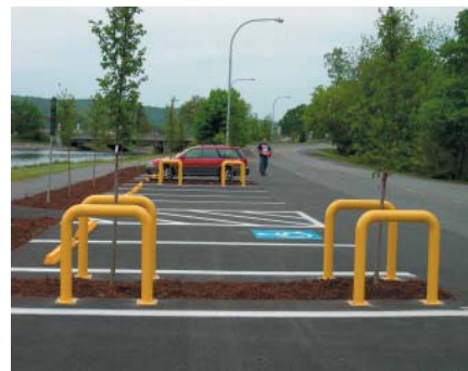
Fig 1.32 Research Parking Lot in Ithaca, N.Y. The foresection is traditional asphalt on CU-Structural Soil® while the back section of the lot is constructed of porous asphalt on CU- Structural Soil®.
