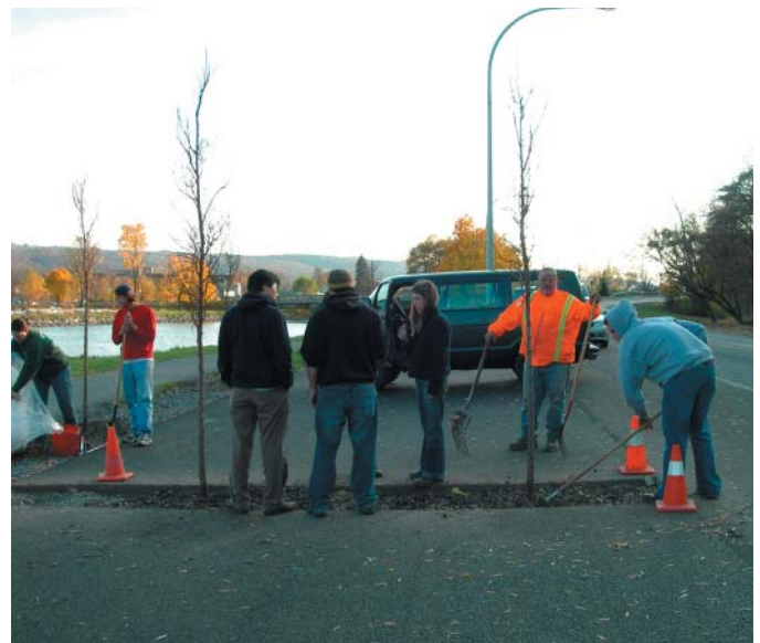
Fig. 1.26 Students planting bare root Ulmus japonica x Ulmus wilsoniana 'Accolade' (Accolade Elm) in the 3' by 18' CU-Structural Soil® tree pit cut into the porous asphalt parking lot in Ithaca, NY in November 2005. 3" of bark mulch was added on top of the CU-Structural Soil®
