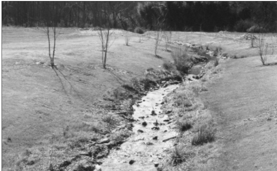
The creek about a year after daylighting. The section in the foreground was previously open, but had its banks regraded; the daylighted section lies in the background. Courtesy of DeKalb County Parks Department.
