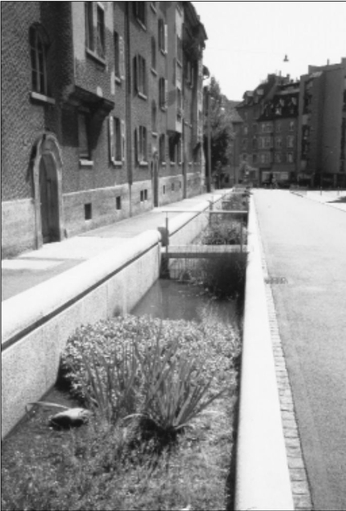
Zürich's engineers daylight brooks and stormwater conduits even in highly built-up portions of the city. Courtesy of Zürich Sewerage Department.
