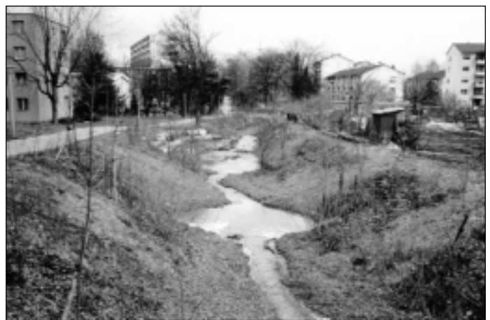
The city of Zürich, Switzerland has daylighted over nine miles of streams and stormwater drainages. These photos show one project before (top) and after. Courtesy of Zürich Sewerage Department.
