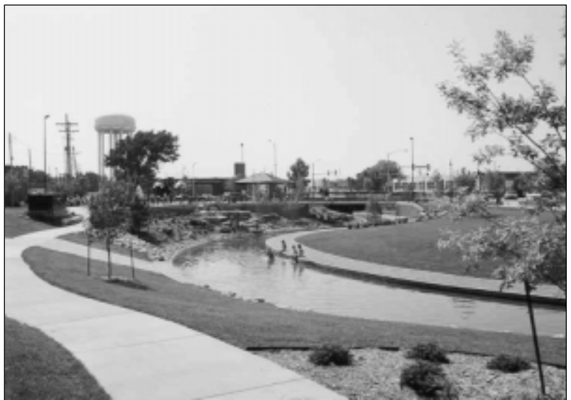
The relocated, daylighted section of Cow Creek in Avenue A Park, Hutchinson, Kansas. Courtesy of City of Hutchinson.
