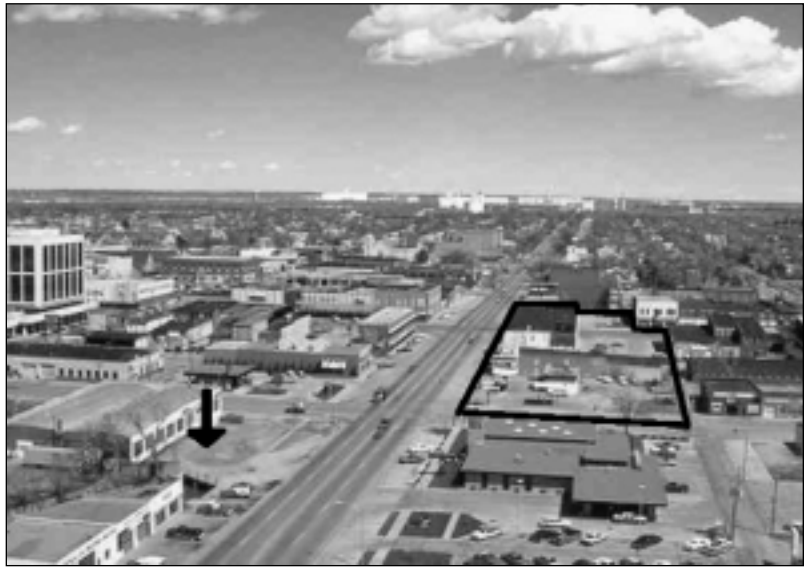
Prior to daylighting, Cow Creek ran underneath much of Avenue A in the center of this photograph. The arrow shows one end of the culvert. The creek was moved to the outlined area and daylighted there in a new park. Courtesy of City of Hutchinson.
