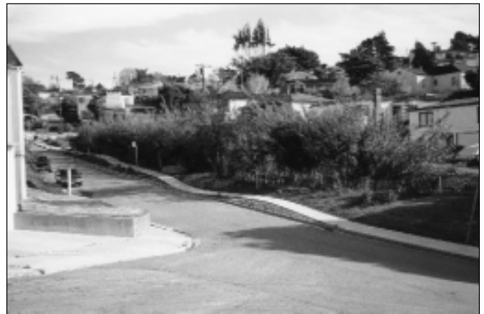
The project in mid-1998, showing the exuberant vegetative growth typical in the early years for projects that stabilize streambanks with bioengineering techniques. Courtesy of Lisa Owens-Viani.
