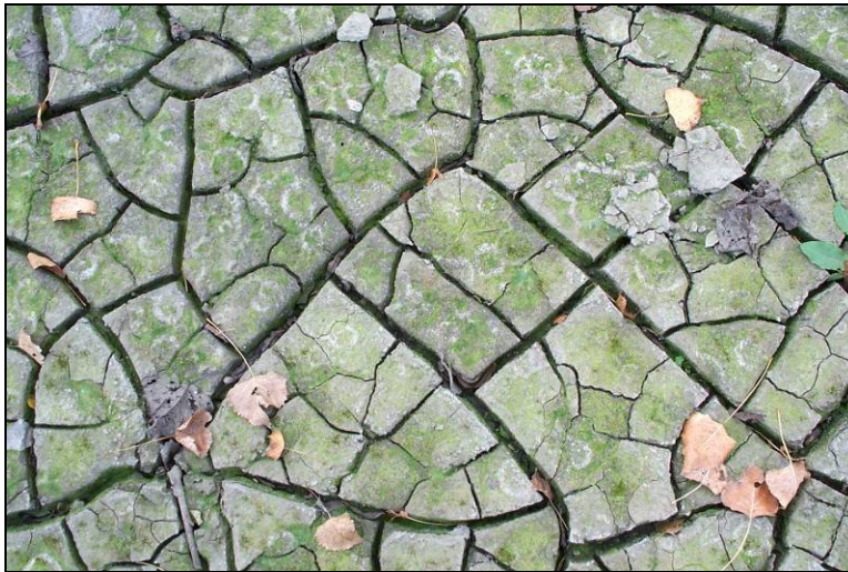
Figure 51. Surface soil cracks in a seasonally ponded depression.
