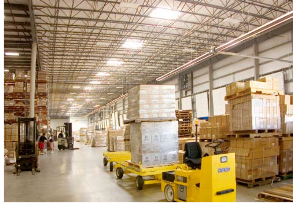
Wide bay, day-lit staging area. Automatic sensors turn off fluorescent fixtures when natural lighting is sufficient.
