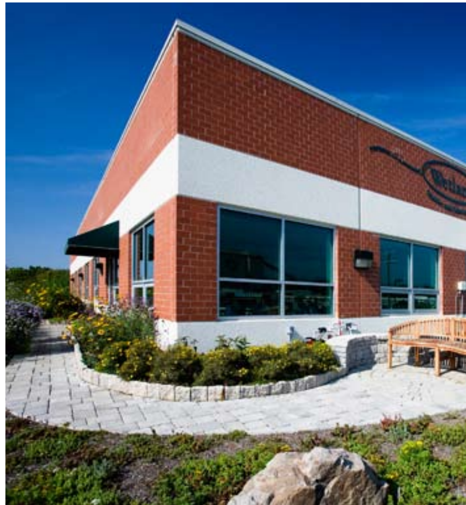
Rear exterior view
