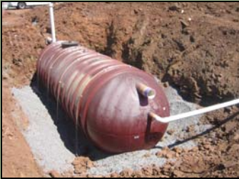
Cistern installation, Sept. 2005
