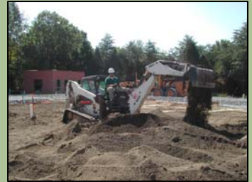
Soil mixing - September 2005
