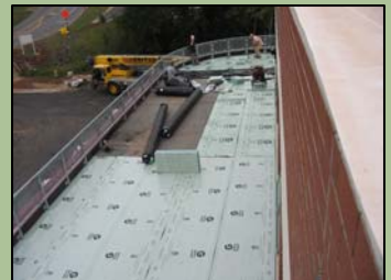
Foam protection board, Oct. 2005
