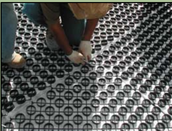
Mat installation, Sept. 2005
