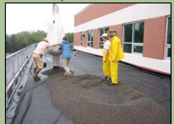
Placing the soil, Oct. 2005
