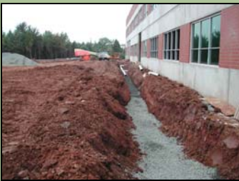
Roof drain trench, Sept. 2005
