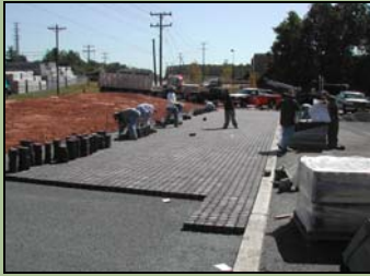
Paver installation, Sept. 2005
