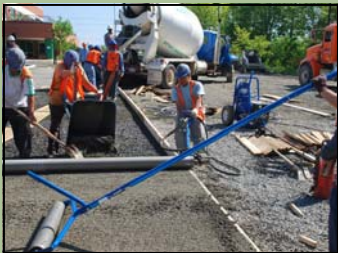
Concrete installation, May 2008
