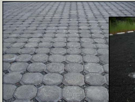
Pervious Concrete Pavers
