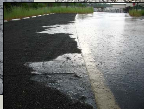
GravelPave2 capturing asphalt runoff
