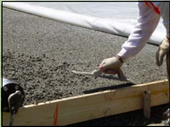
Concrete installation, May 2008
